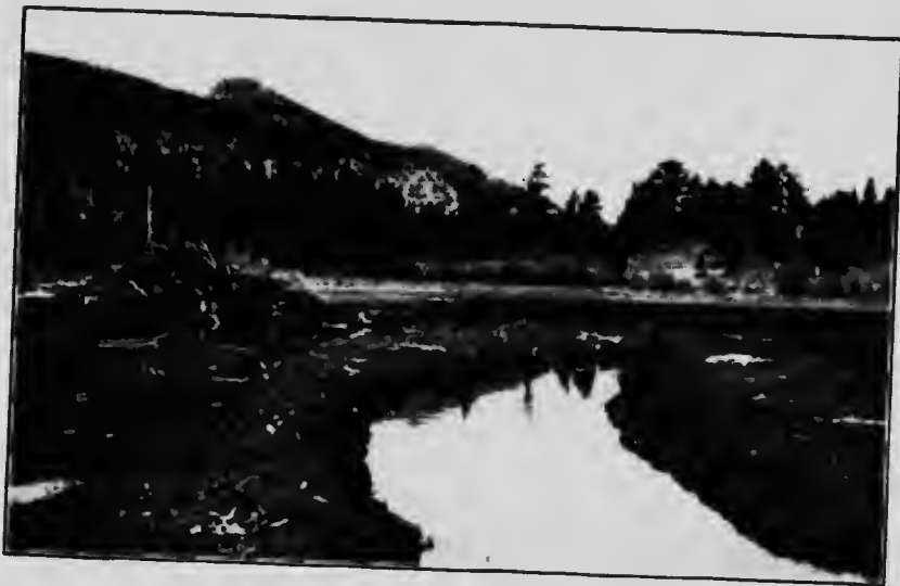
SECTION OF A 750-FOOT CANAL AT LILY LAKE Here five feet wide and three feet deep
